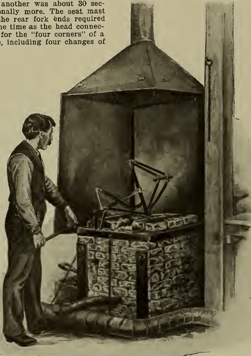
Dipping the Bottom Bracket—Front View of Fulton Furnace.
